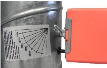
The minimum position screw can also be used to determine the damper position. The setscrew is aligned with the position of the damper blades. When the setscrew is in line with the duct, pointed at the Closed on the minimum position label, the damper is actually open. When it is hidden behind the motor and stopped against the anti-rotation post on the motor, it is Closed or at the minimum position.
